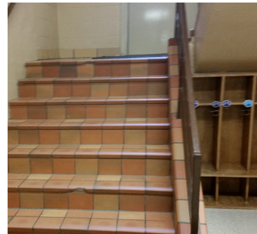
Ceramic tile in stairwells
