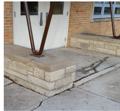
Exit landing and walk cracks
