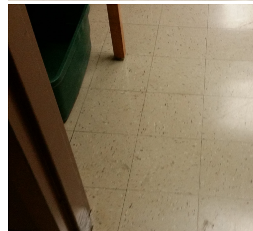
Classroom VAT tile
