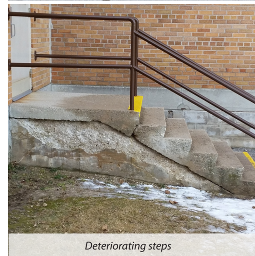
Exit landing and walk cracks
