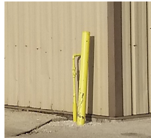
Cracked bollard base
