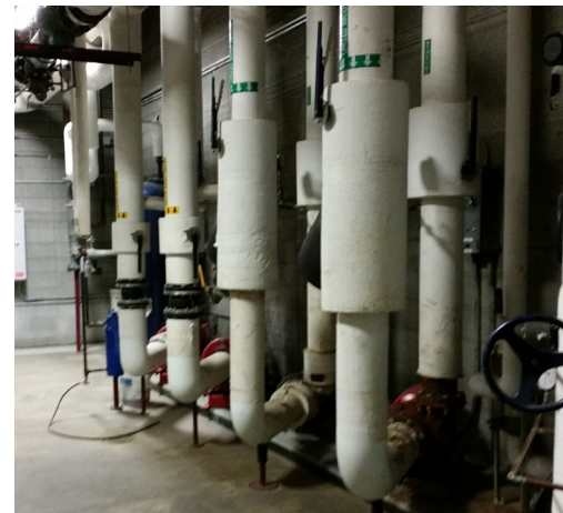
Variable volume hot water heating pumps
