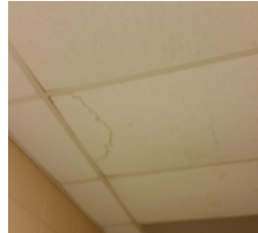
Ceiling tile and discolored suspension grid
