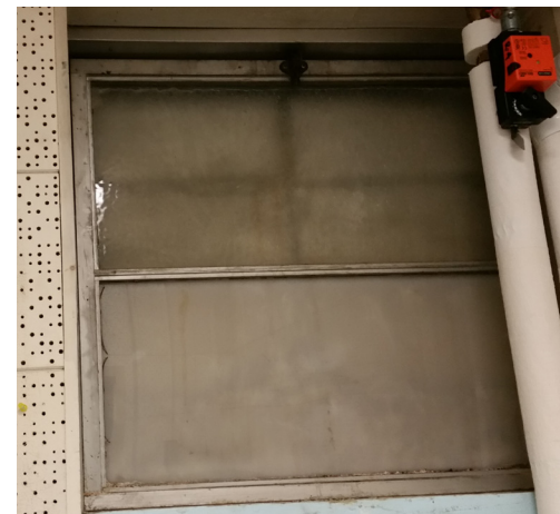
Covered Glass Block Window
