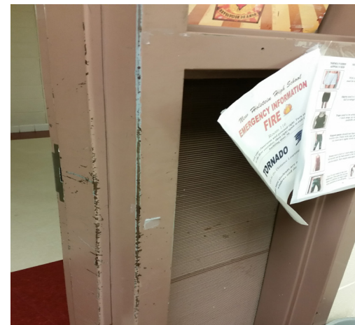
Classroom door frame
