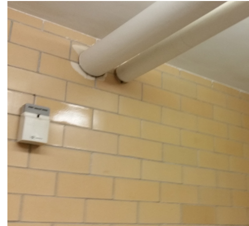
Exposed pipes and penetrations
