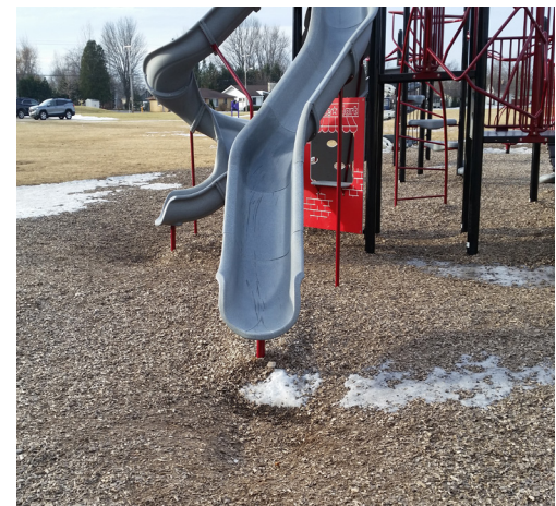
Compressed fall surface under slide
