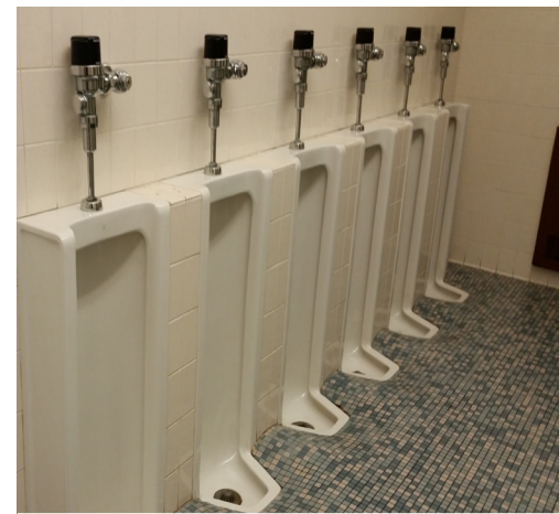
High school floor tiles
