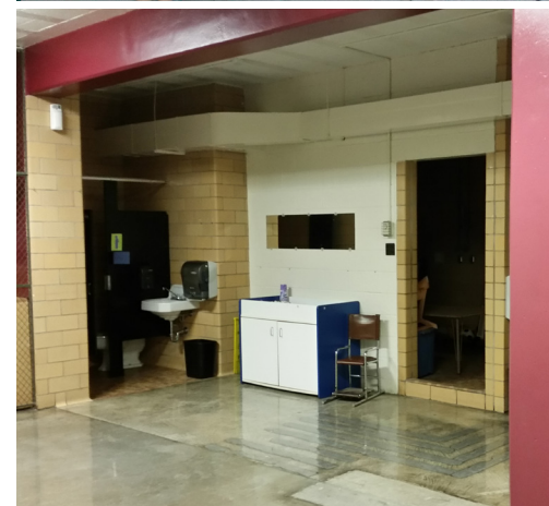
Existing locker room area
