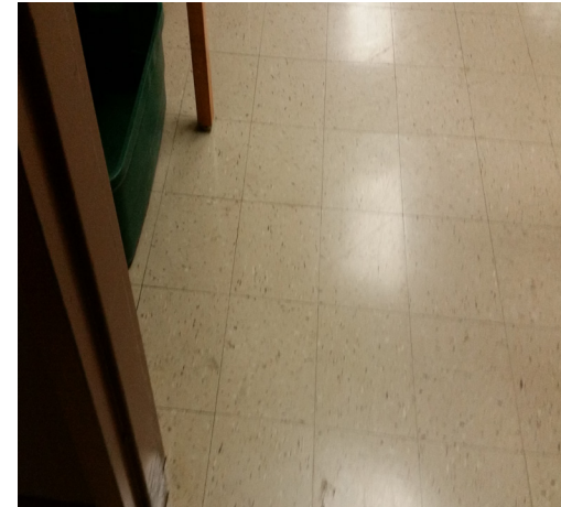
Classroom VAT tile
