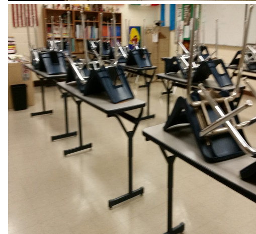
Classroom VAT tile
